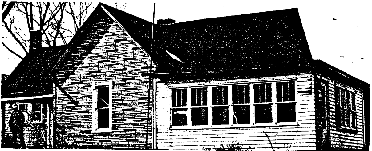
Figure 21.—Test structure 27, near a coal mine.
