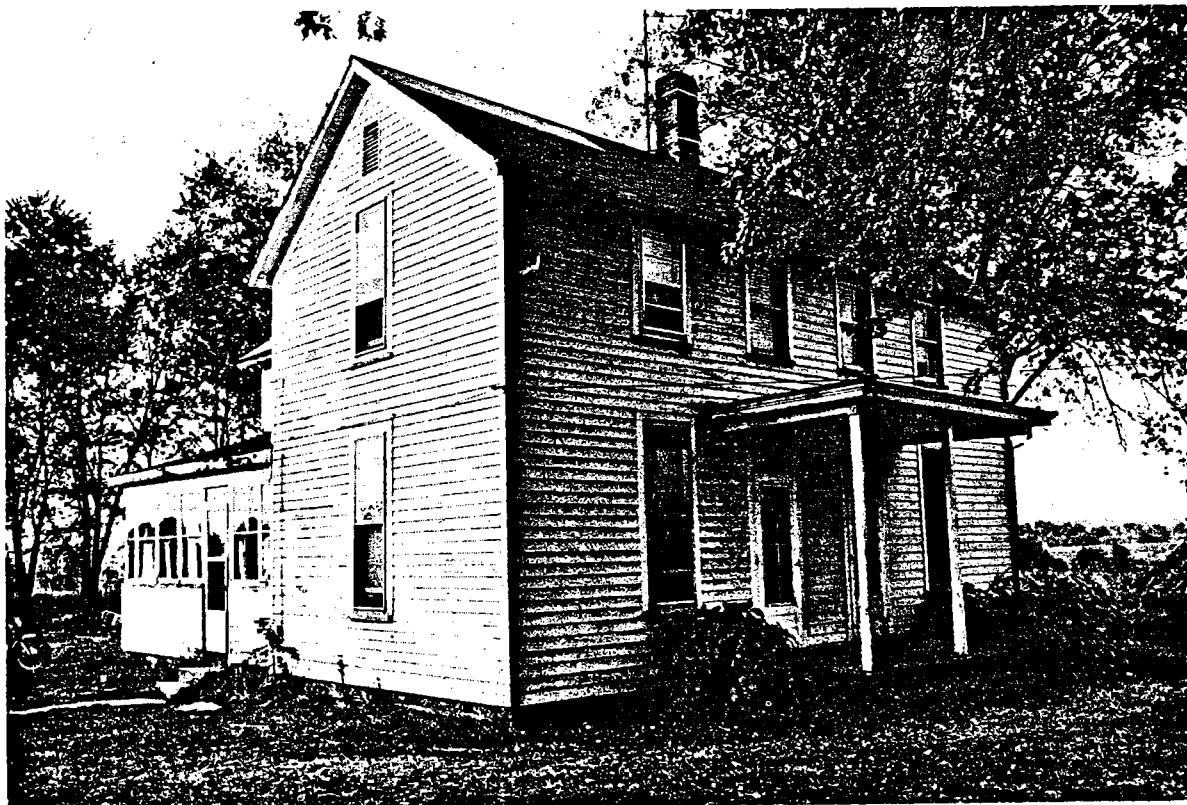
Figure 15.—Test structure 19, near a coal mine.
