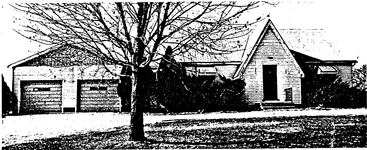
Figure 16.—Test structure 20, near a coal mine.
