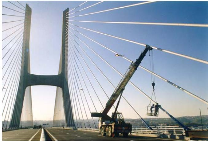
**FIG. 13. Installation of accelerometers on stay cables**
