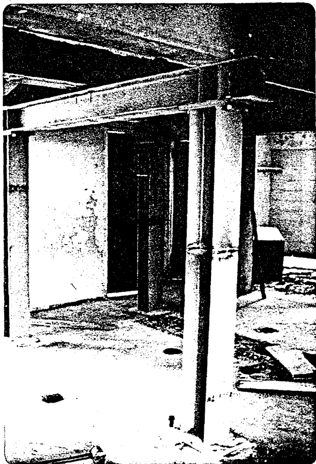
Fig. 54 Cribbing, 10 th Floor
