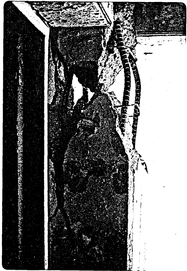
Fig. 97 Col. 38, 4 th Floor After Completion of Testing
