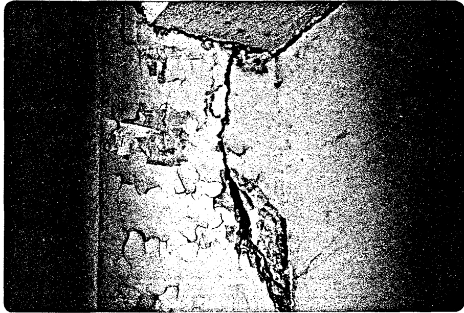
Fig. 70 Top of Col. 37 in the Second Story, After E.W. Shaking
