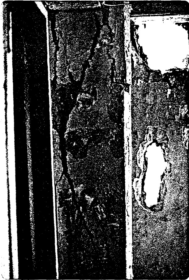
Fig. 96 Col. 38, 4 th Floor Prior to Last Shaking
