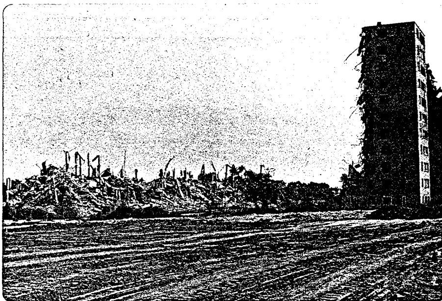
Fig. 6 Pruitt-Igoe Buildings During Demolition
