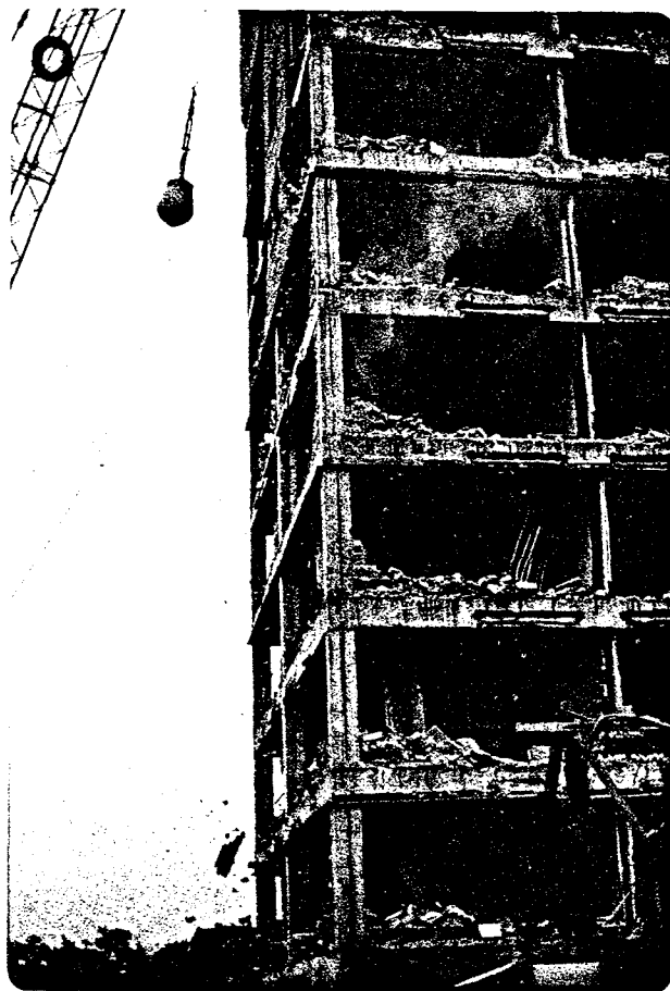
Fig. 27 Removal of Walls after E.W. Shaking
