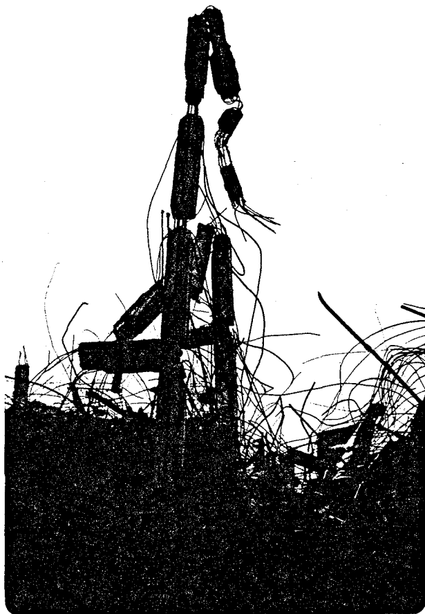
Fig. 9 A Former Corner Column During Demolition
