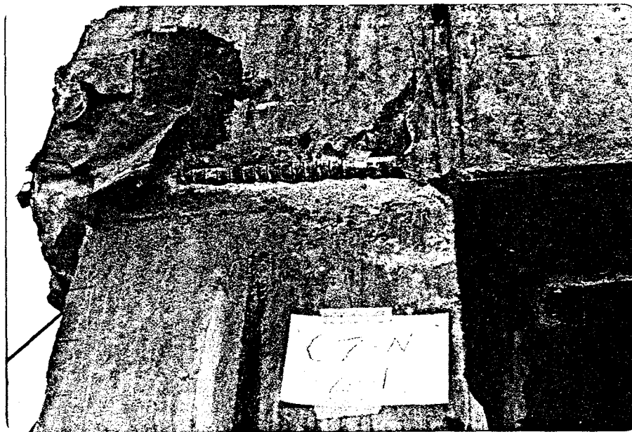
Fig. 74 Exposed Reinforcing Bar, After E.W. Shaking
