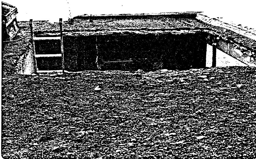
Fig. 21 Opening in Roof
